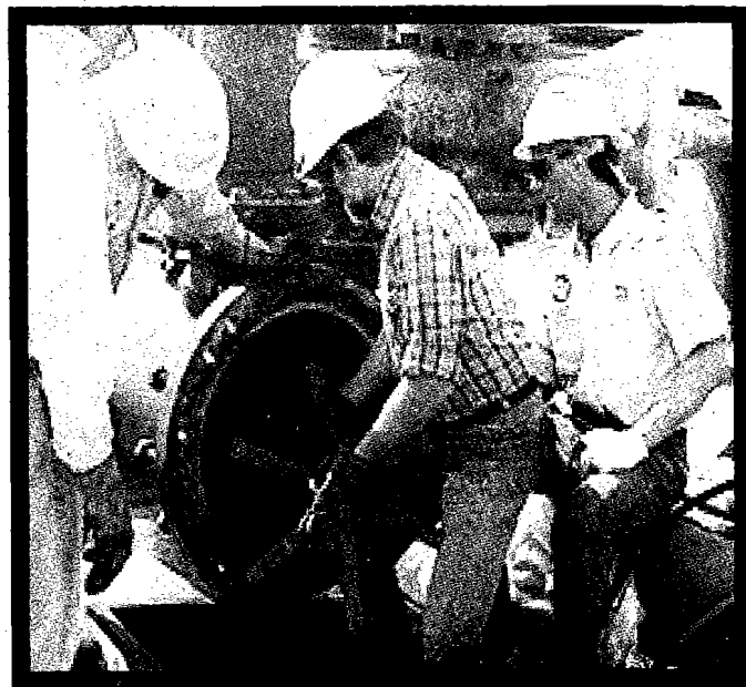
Photo #3. Pig tracker being attached to the tool in the launch tube prior to closing up the launcher and beginning a cleaning run.
