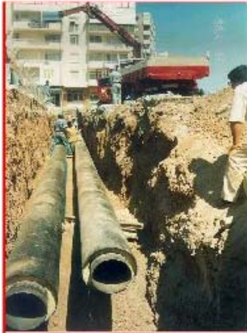
Figure 2: Pre-Insulated Steel Pipes (Casing is FRP) for geothermal heating network distribution
